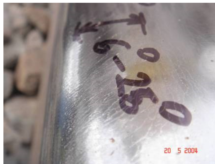
Moderate checking at the gauge corner of the rail.
