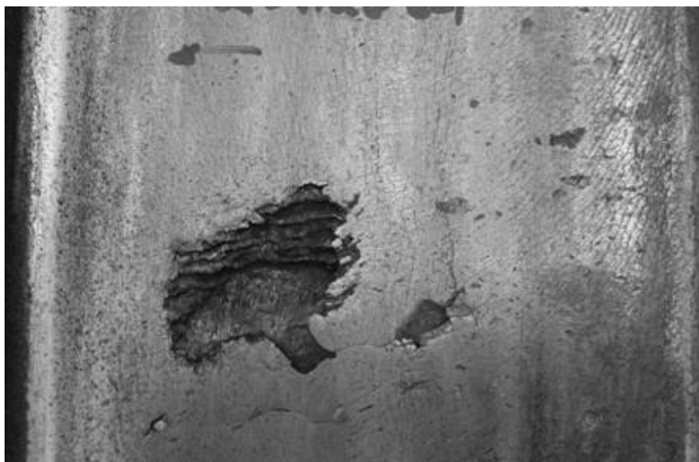
Continued propagation of cracks into the wheel surface leads to tread shelling.
